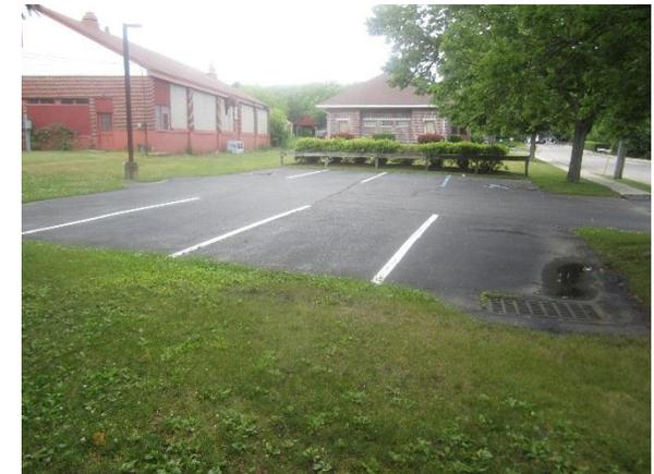
Stormwater is currently directed to an existing catch basin and the local sewer system. Parking spots in both the south and the north parking lot can be replaced with porous asphalt to capture and infiltrate stormwater. A rain garden adjacent to the building can capture, treat, and infiltrate roof runoff. A preliminary soil assessment suggests that the soils have suitable drainage characteristics for green infrastructure.
