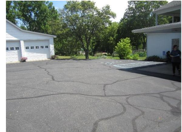
Stormwater currently flows across the parking lot. Parking spots adjacent to the south building can be replaced with porous asphalt to capture and infiltrate stormwater. A preliminary soil assessment suggests that the soils have suitable drainage characteristics for green infrastructure.
