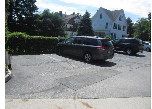
Stormwater is currently directed to the local sewer system through connected downspouts or existing catch basins. Parking spots on the east side of the building can be replaced with porous asphalt to capture and infiltrate stormwater. Rain gardens on the front lawn of the building can capture, treat, and infiltrate roof runoff. A preliminary soil assessment suggests that the soils have suitable drainage characteristics for green infrastructure.
