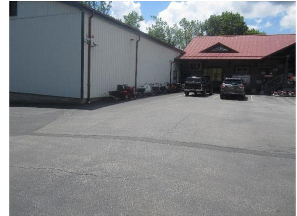
Stormwater is currently directed to the local sewer system by connected downspouts. A cistern can be installed on the south building to capture roof runoff. The water can then be used for washing vehicles or for other non-potable uses. A preliminary soil assessment suggests that the soils have suitable drainage characteristics for green infrastructure.
