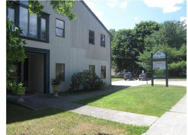
Stormwater is directed to the ground by disconnected downspouts. A rain garden adjacent to the building can capture, treat, and infiltrate roof runoff. A preliminary soil assessment suggests that the soils have suitable drainage characteristics for green infrastructure.
