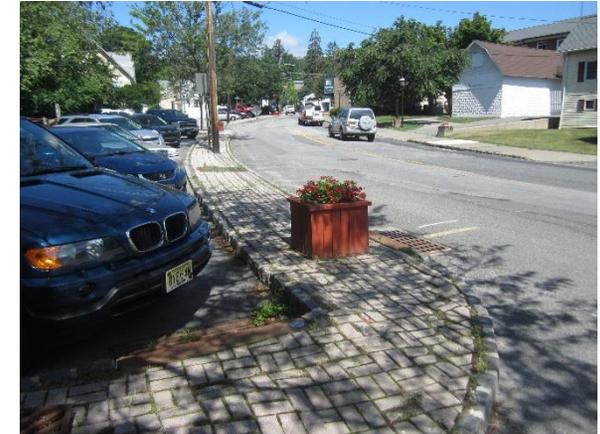
Stormwater is currently directed to an existing catch basin. Parking spots on the north side of the lot can be replaced with porous asphalt to capture and infiltrate stormwater. A preliminary soil assessment suggests that the soils have suitable drainage characteristics for green infrastructure.
